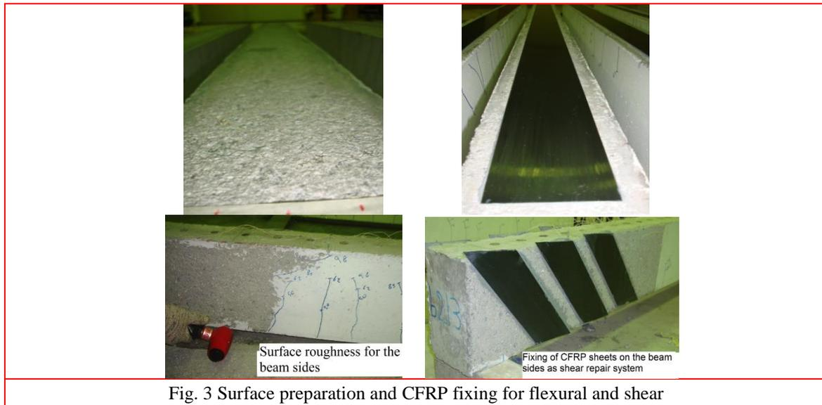
Fig. 3 Surface preparation and CFRP fixing for flexural and shear
