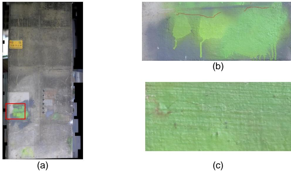
Fig. 3. Example of Damage Detection using the Proposed System in a Real Structure: (a) Bridge Pier Image, (b) Concrete Damage Detection Result (Red area denotes crack area) and (c) Image of the area with crack detection
