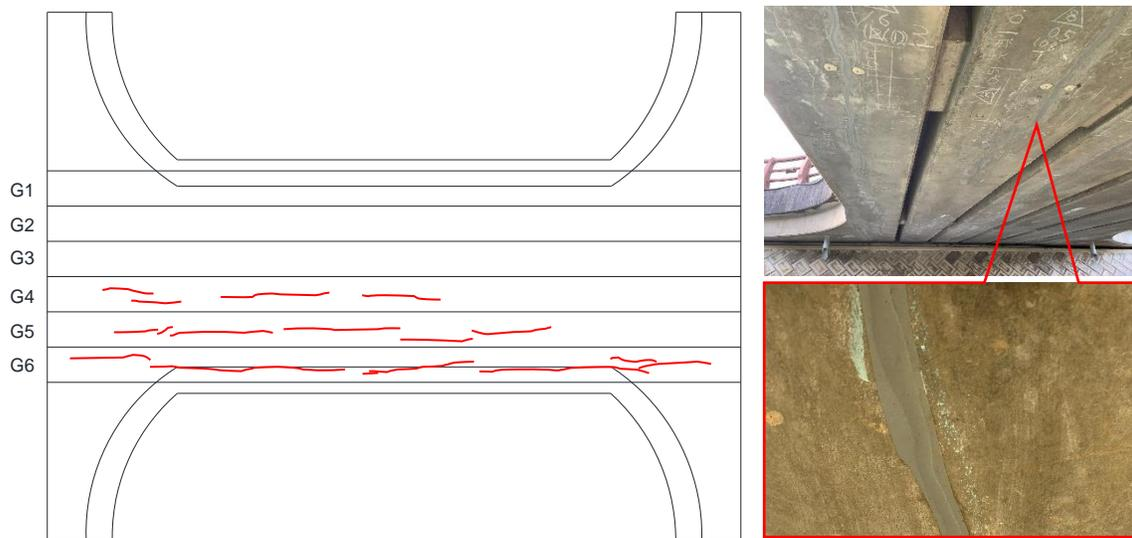
**Fig. 3** Measured cracks positions and patterns on the girders
