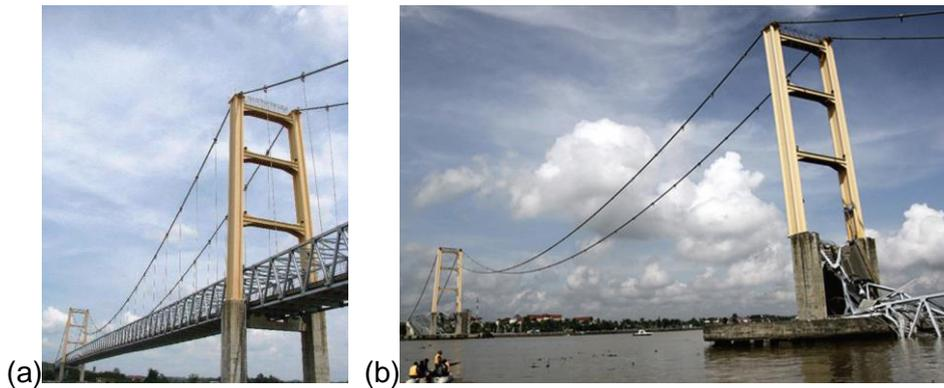
**Fig. 1** Collapse of the Kutai Kartanegara Bridge: (a) before collapse (b) after collapse
