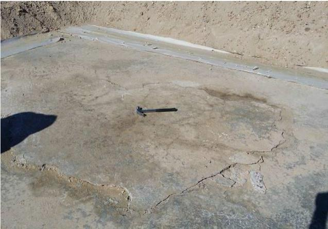
Fig. 6. Concrete spalling due to reinforcement corrosion in one of the severely damaged reservoirs.
