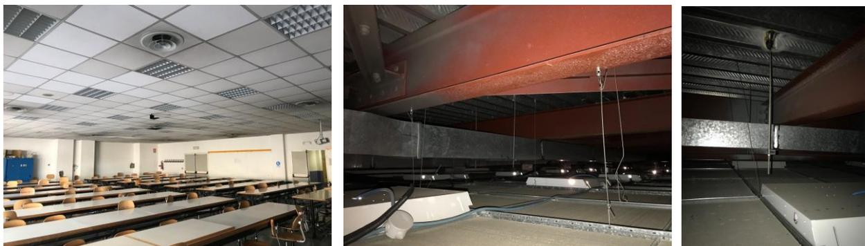
**Fig. 1** Some pictures of the suspended ceiling
