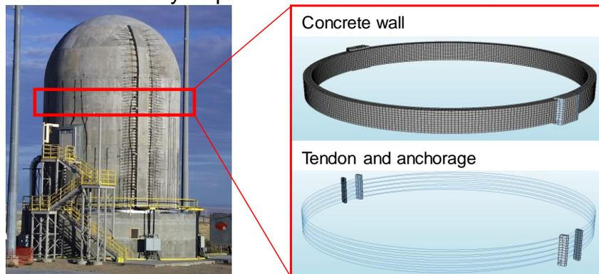
Fig. 2 Original experiment specimen (Hessheimer et al., 2003) and numerical model
