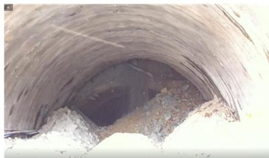
Fig. 1 Collapse of tunnel in a large-scale fault clay zone
