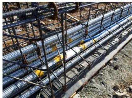
Fig. 1 Installation of embeddable EM sensor
