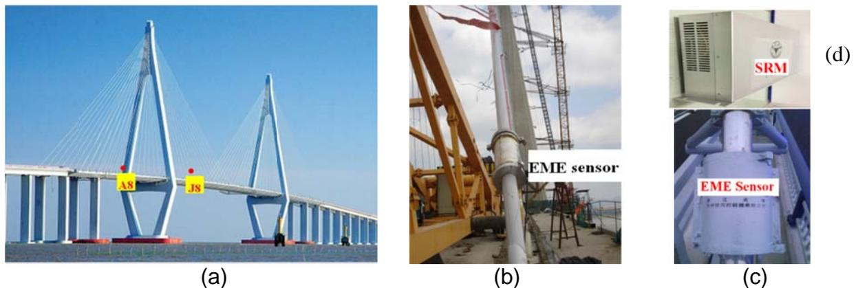
Fig. 4 Stress monitoring in the Second Jiaojiang Bridge. (a) The Second Jiaojiang Bridge, (b) EME sensor during the construction, (c) EME sensor for long-term monitoring, and (d) The signal regulating module (SRM).
